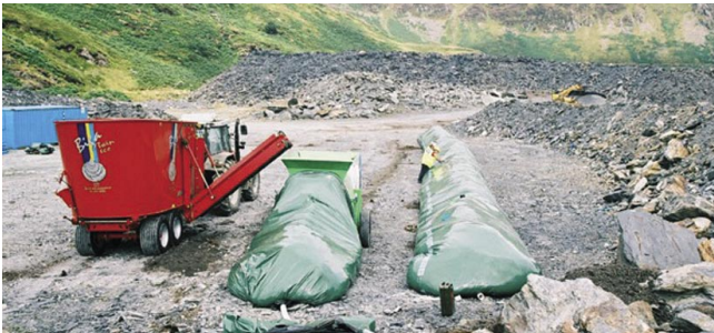
Producing compost to revegetate slate waste tips in Wales.
